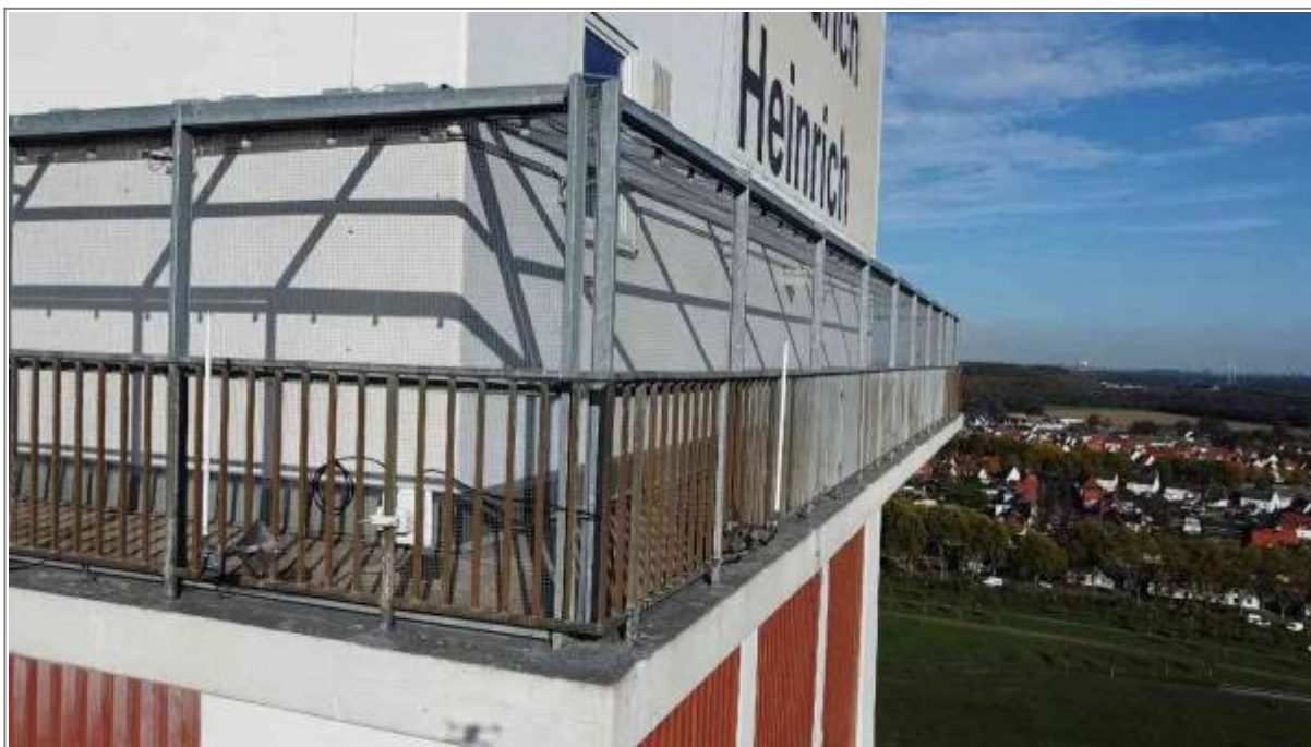
Fig.: The two white rod antennas at the southwest corner of the tower of the Friedrich-Heinrich colliery.
