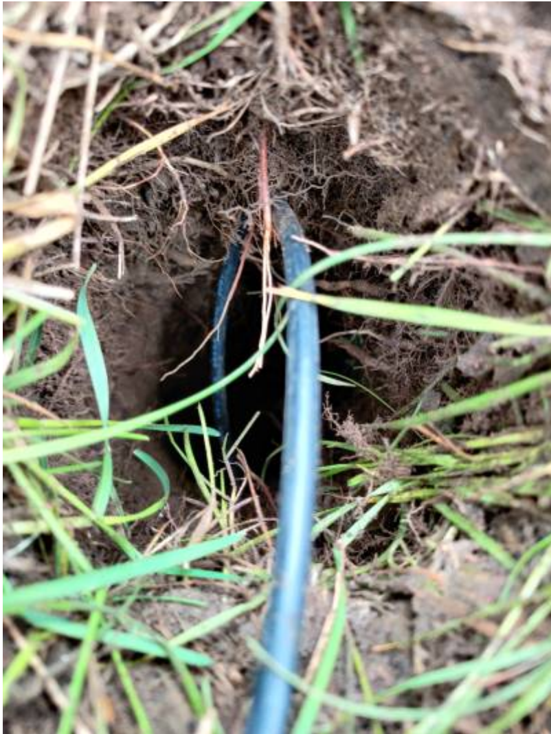
The sensor is installed in a 30cm deep hole.
