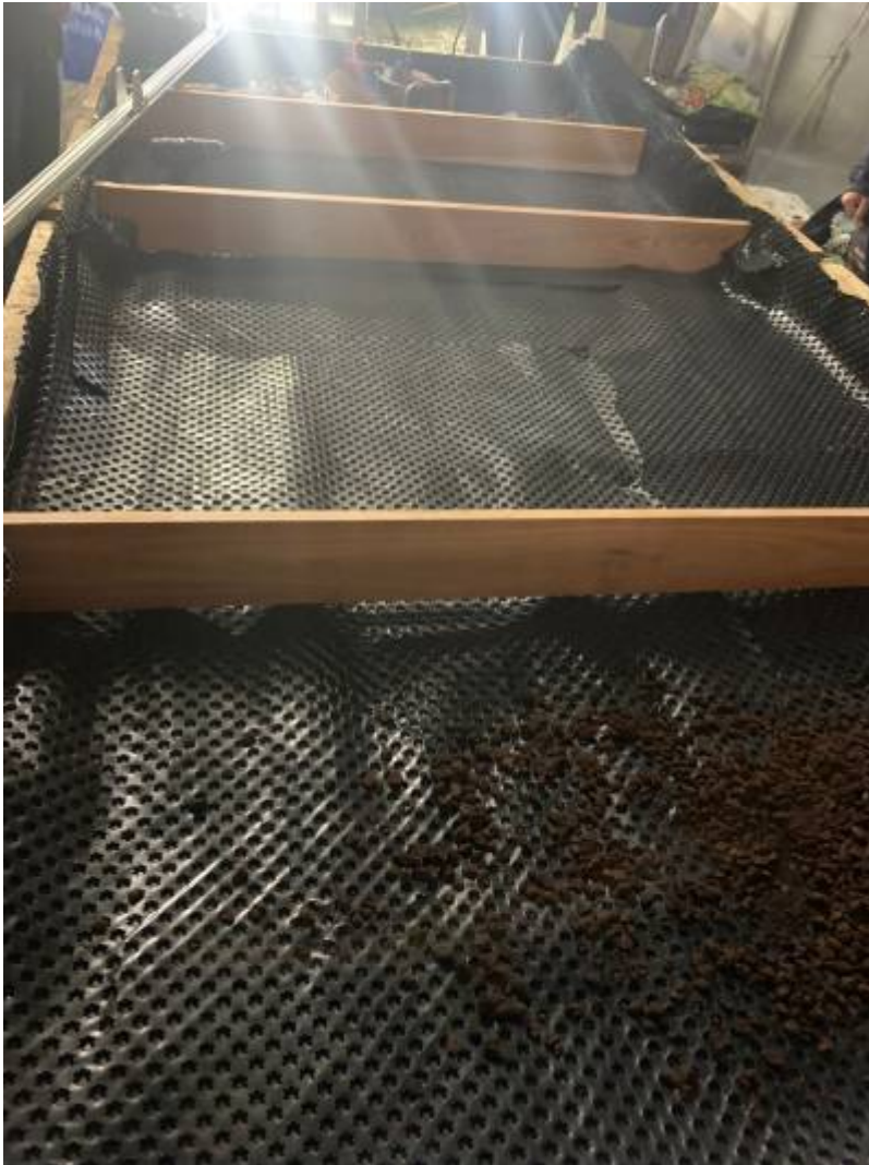
Fig - 5 Installation of drainage net and dividers
