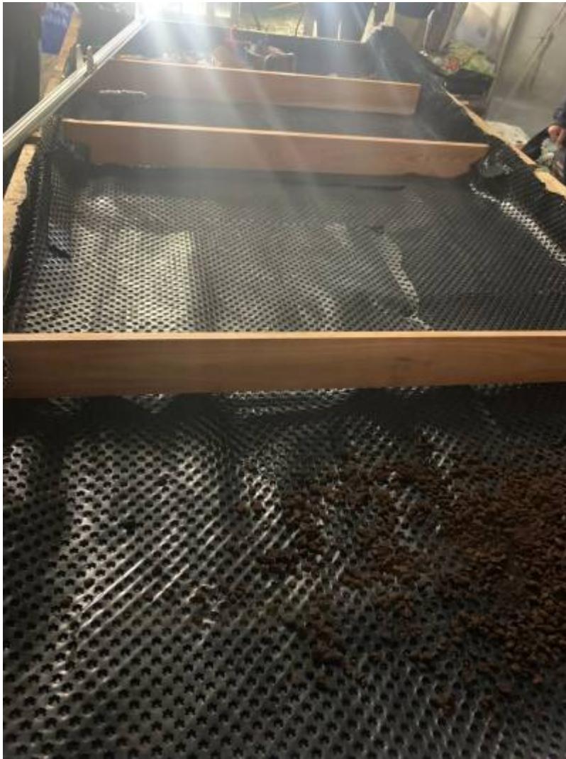
Fig - 5 Installation of drainage net and dividers
