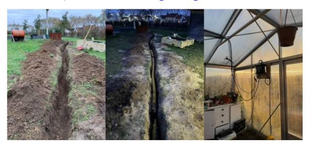
The next was to establish a water connect with an inlet at the water source which was just beside the one for electricity, and an outlet in the greenhouse. Both were linked with a simple pipe equipped
