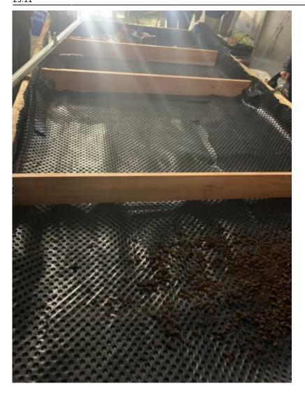
Fig - 5 Installation of drainage net and dividers
