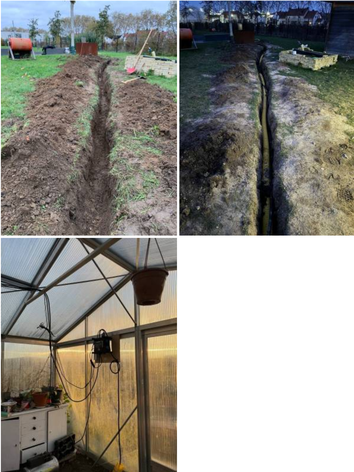
Fig - 8 Pictures of the Trench before the pipe (Left), after the pipe (middle) and the electrical hub (right)
