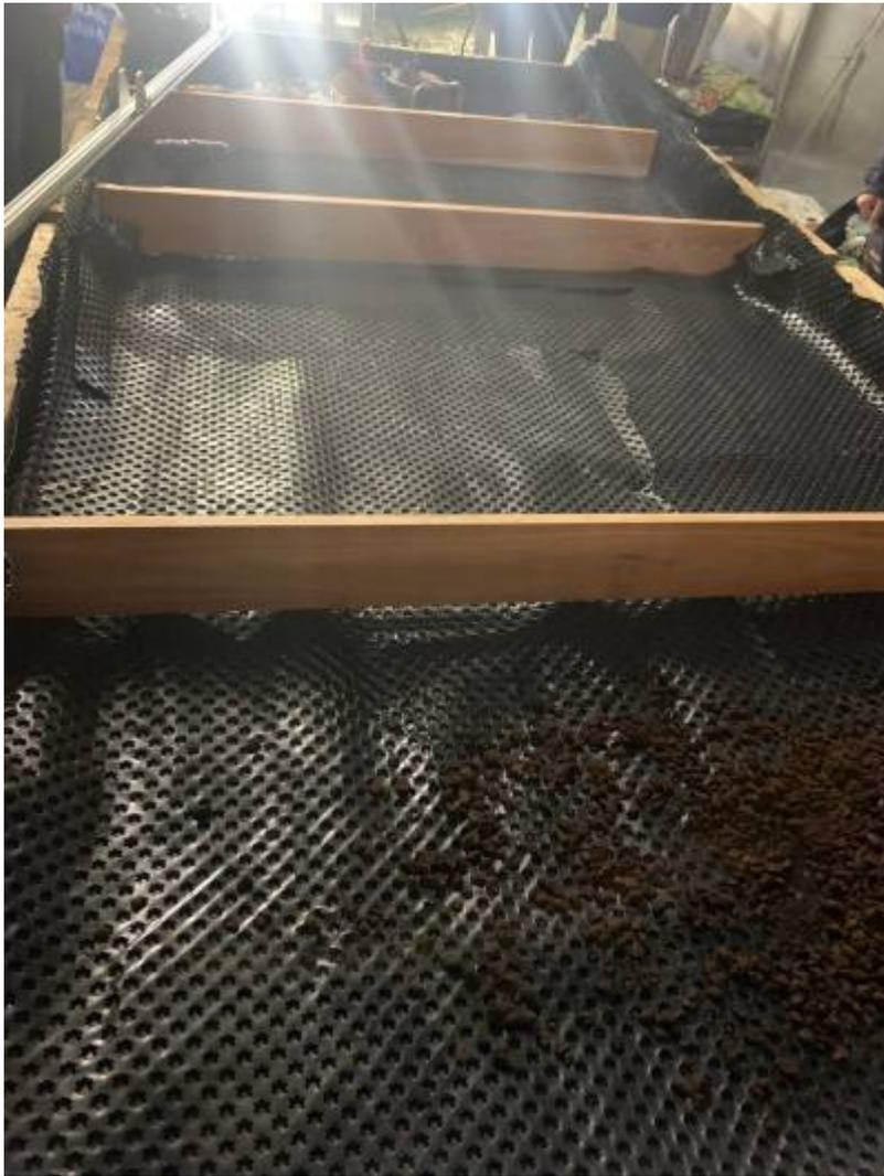
Fig - 5 Installation of drainage net and dividers
