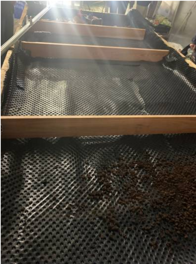
Fig - 5 Installation of drainage net and dividers
